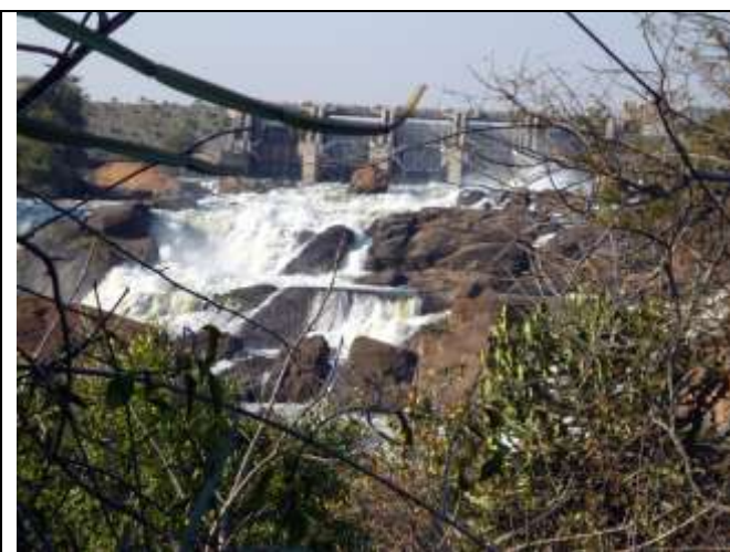
Hamilton Falls, harnessed as power station
